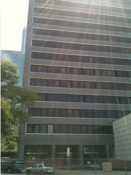
Figure 1: Exterior View West
